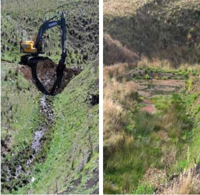
*Establishment of weirs on Gunningrah has lead to significant gully restoration in as little as two years - 2006 (left), 2008 (right)*
