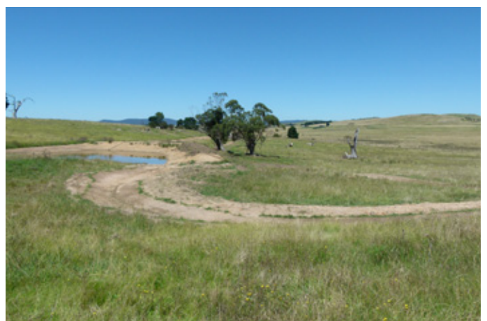
Contour channels spread water across the property
