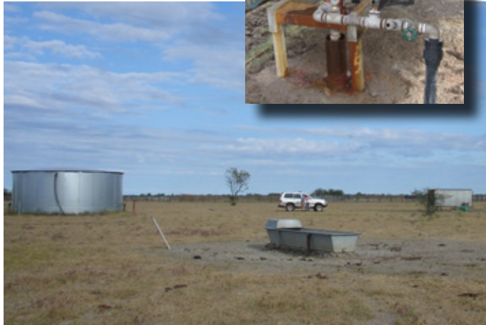
Water infrastructure now comprises a network of steel or plastic storage tanks, concrete or steel troughs and bores Inset: A diesel bore pump
